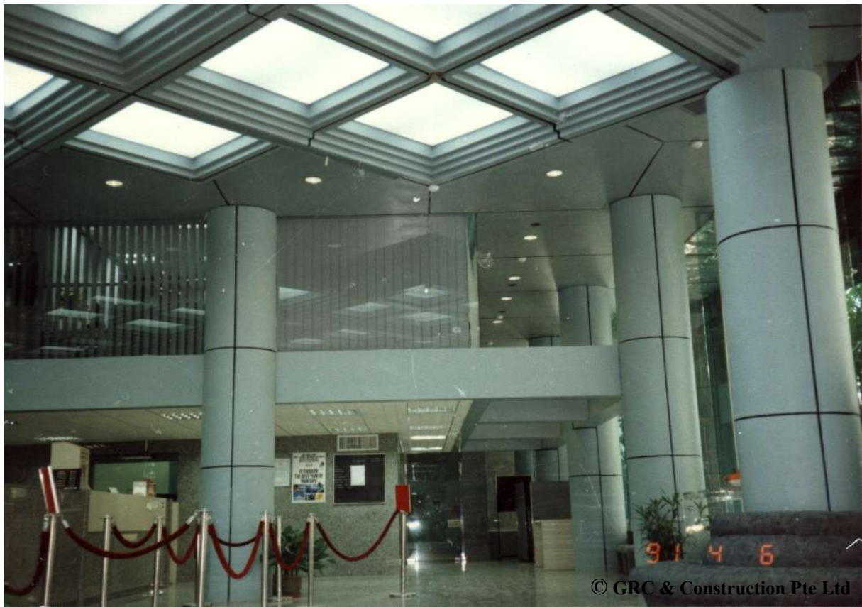
A & A WORKS TO MALAYAN BANKING BERHAD AT BATTERY ROAD GFRC FALSE COLUMNS & SUSPENDED CEILINGS
