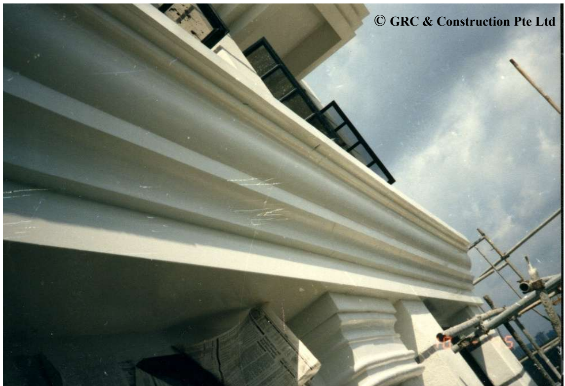
PINEWOOD GARDEN CONDOMINIUM GFRC CORNICE TO EXT.FACADE
