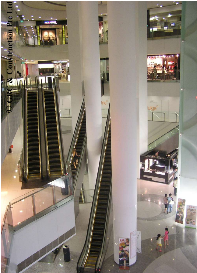
CENTRAL @ CLARKE QUAY GRG SQUARE & CIRCULAR COLUMN CLADDING
