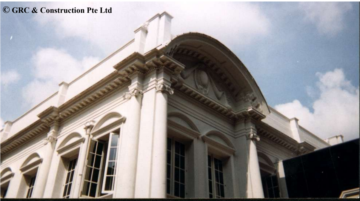
PARLIAMENT COMPLEX AT NORTH BRIDGE ROAD GFRG DECORATIVE FEATURES/PEDIMENT/COLUMN/ENTABLATURE
