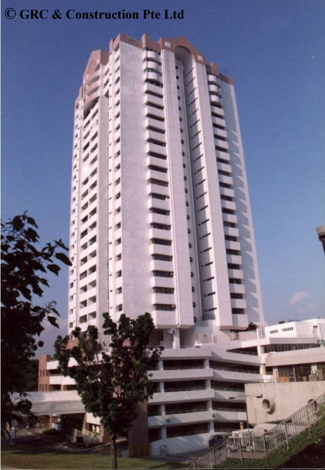
A&A WORKS AT BEAUTY WORLD CENTRE GFRG DECORATIVE ROOF, WALL CLADDING
