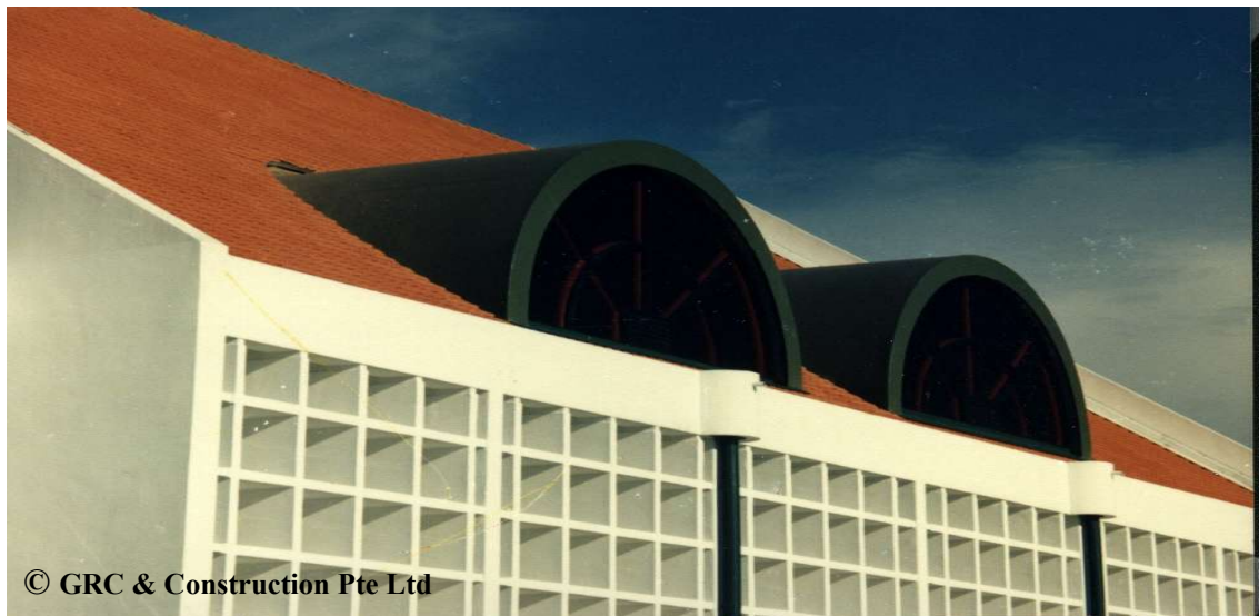
RAFFLES INSTITUTION AT BISHAN STREET 11 GFRC ROOF & PRECAST CONCRETE FINS
