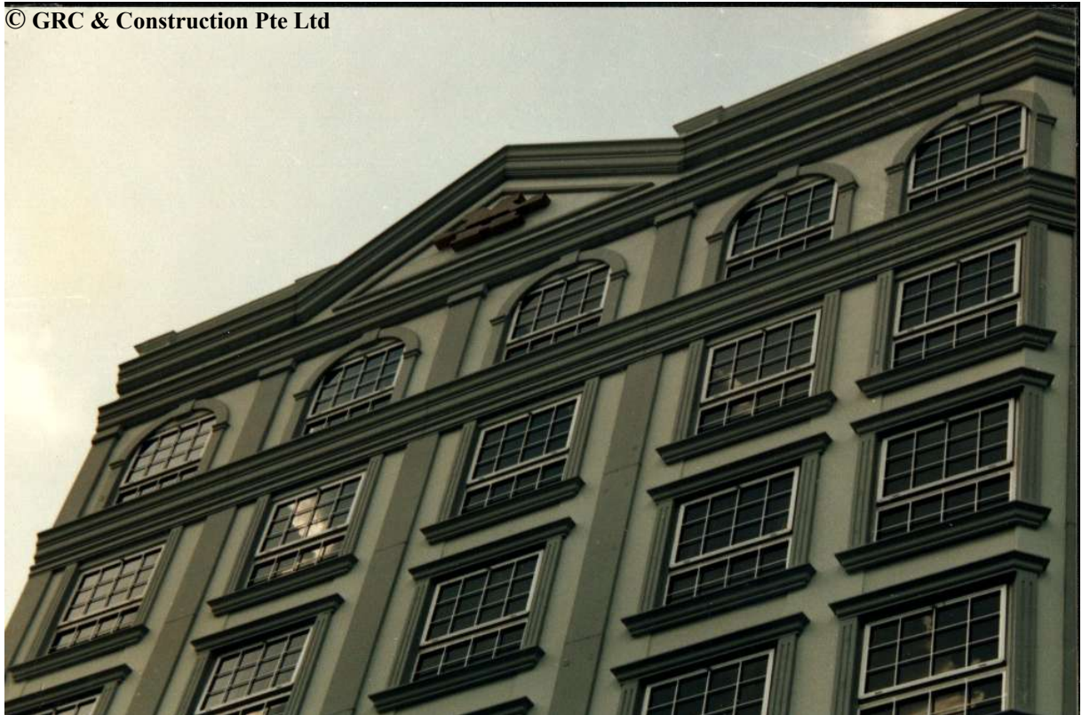
METROPOLE HOTEL AT SEAH STREET GRC CORNICES, COLUMN CLADDINGS & MOTIFS
