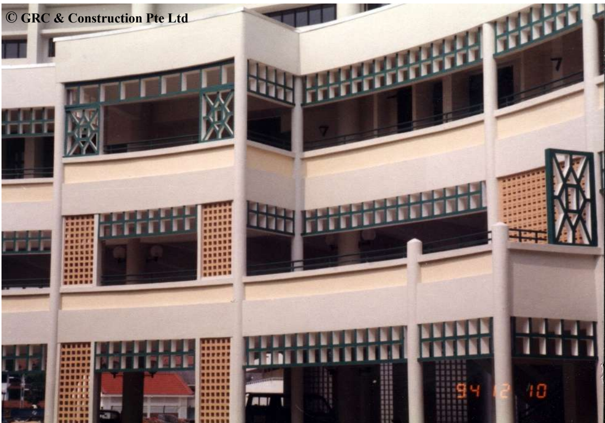
TANJONG KATONG GIRLS SCHOOL GFRC SUNBREAKERS
