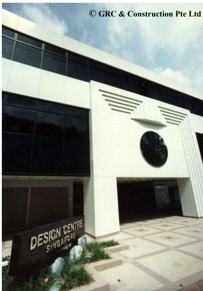
DESIGN CENTRE AT NO. 141 NORTH BRIDGE ROAD GFRC EXT. WALL CLADDING & GLAZING WORK
